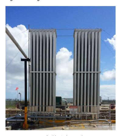
Figure 4. Ambient air vaporizers
