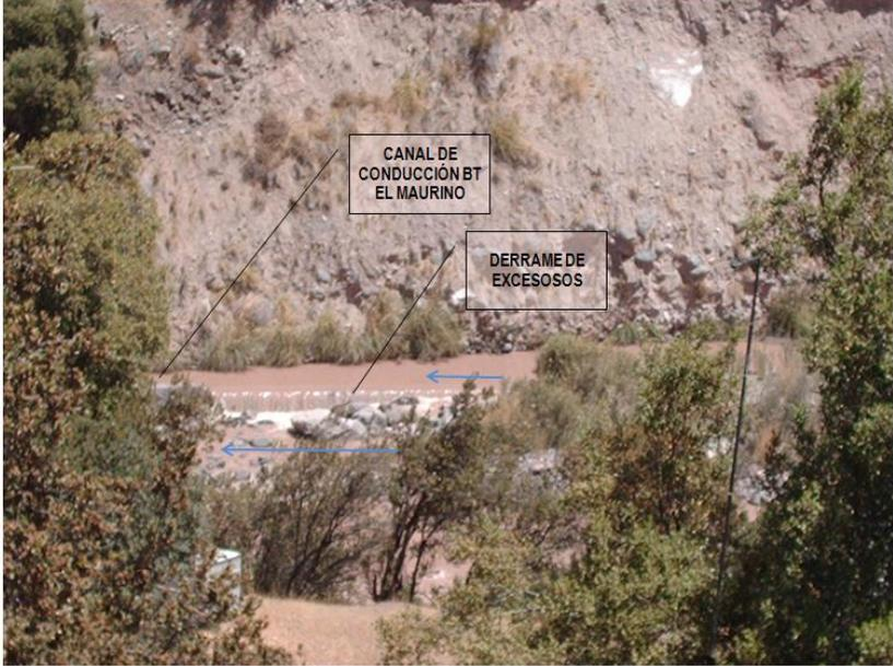
The photograph shows a rocky, steep hillside with a concrete canal structure. Two blue arrows point to the canal, and two black arrows point to an overflow area. The text 'CANAL DE CONDUCCIÓN BT EL MAURINO' is in a box with a black arrow pointing to the canal. The text 'DERRAME DE EXCESOS' is in a box with a black arrow pointing to the overflow area.
